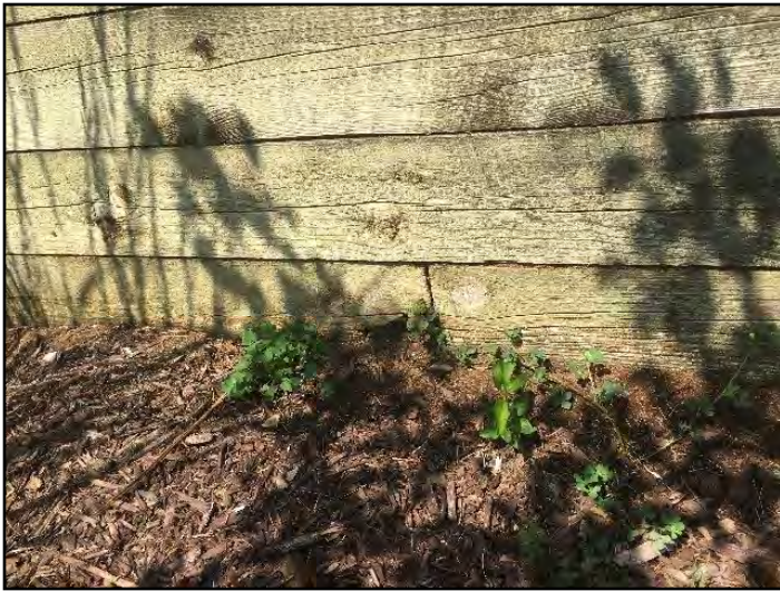
26. Rot or insect damage
