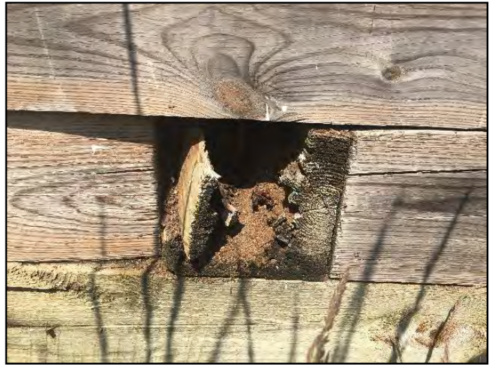
27. Rot or insect damage
