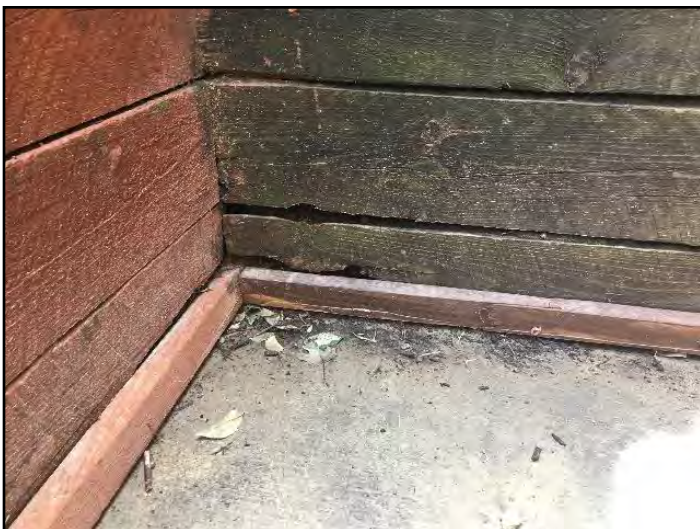
32. Rot or insect damage
