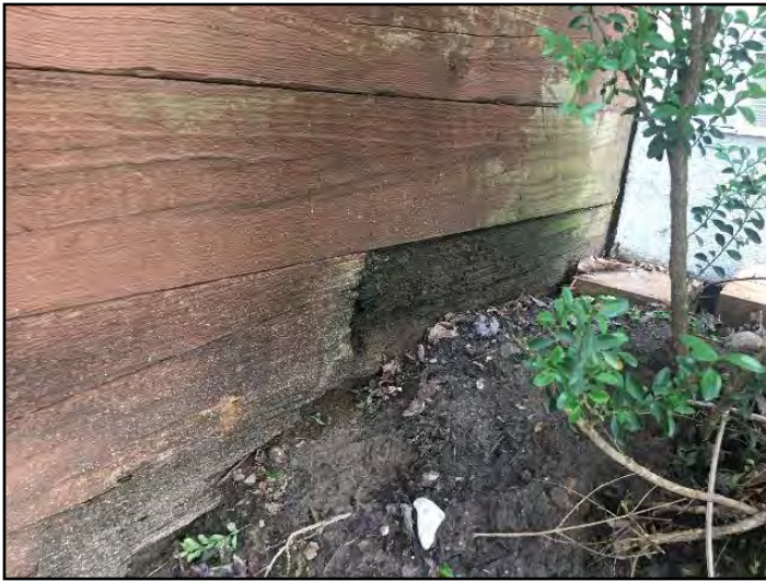
30. Rot or insect damage
