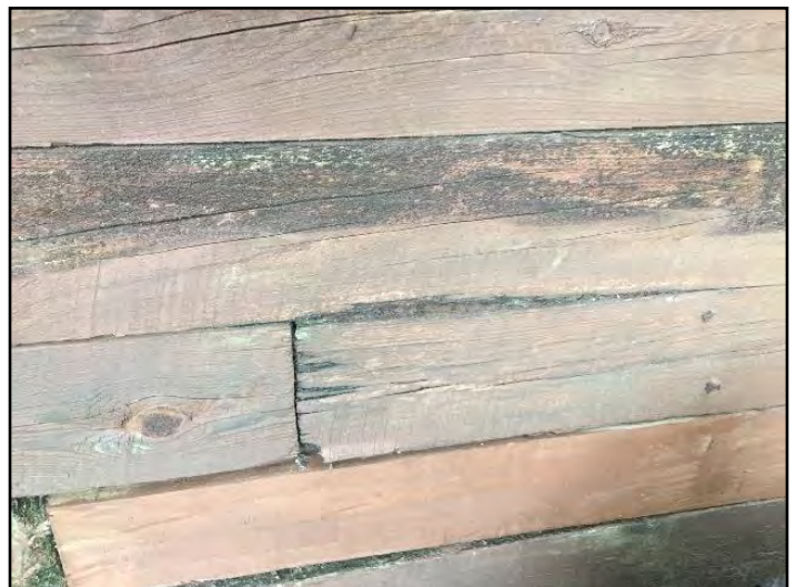
29. Rot or insect damage
