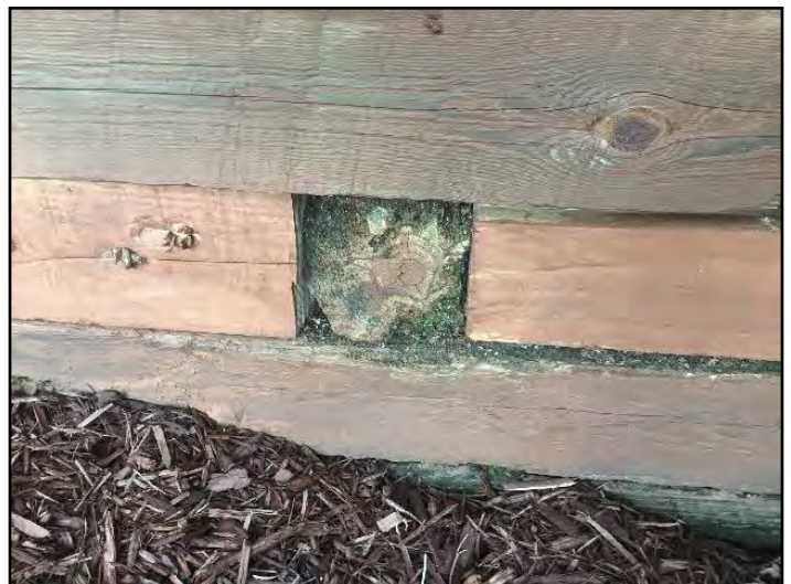
33. Rot or insect damage
